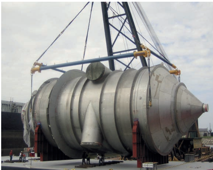
A 127-tonne flue-gas scrubber tower being prepared for installation
