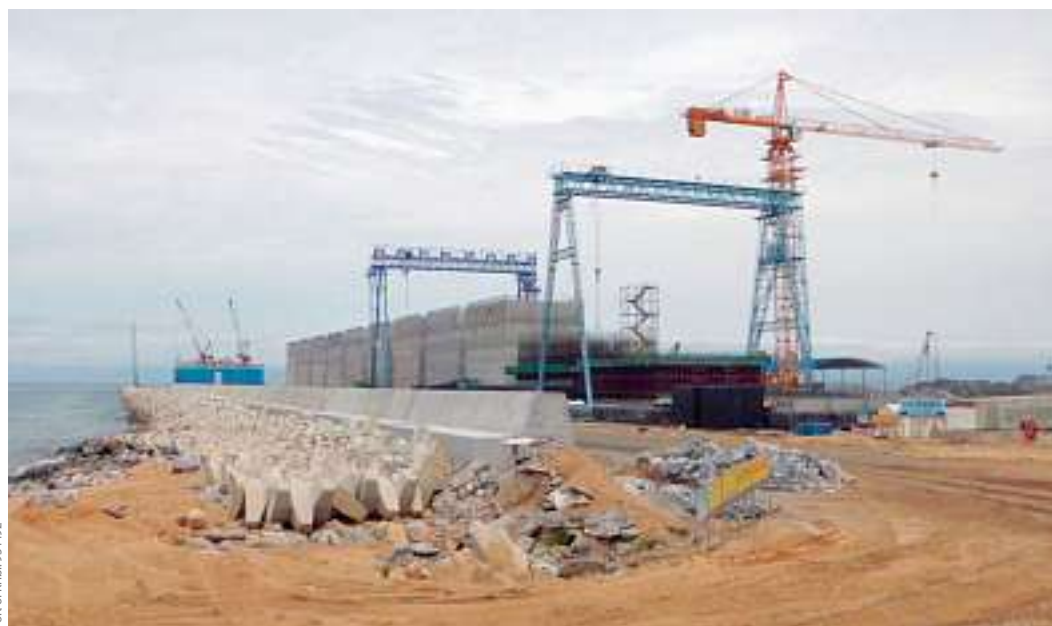
Port of Kribi's breakwater under construction
