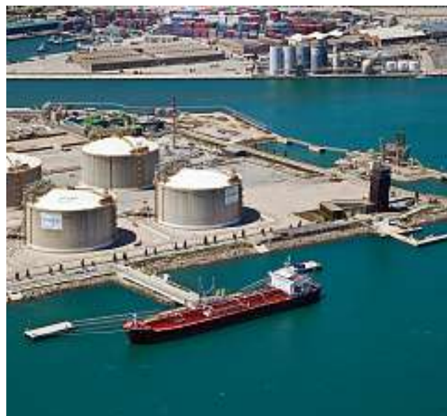
The Port of Barcelona is home to Europe's oldest regasification plant, owned by Enagas
