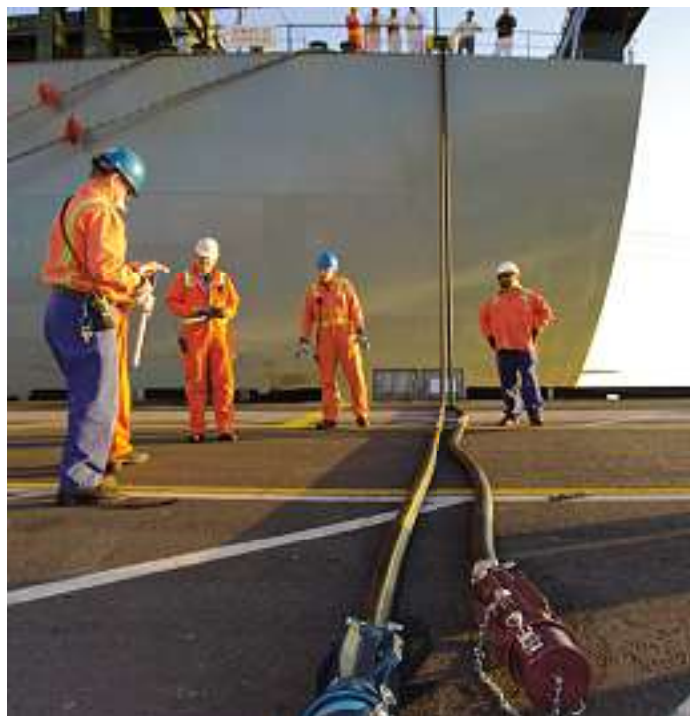
OPS connection at Port of Long Beach, USA. Some European ports are opting for high-voltage systems, whilst others are choosing low-voltage
