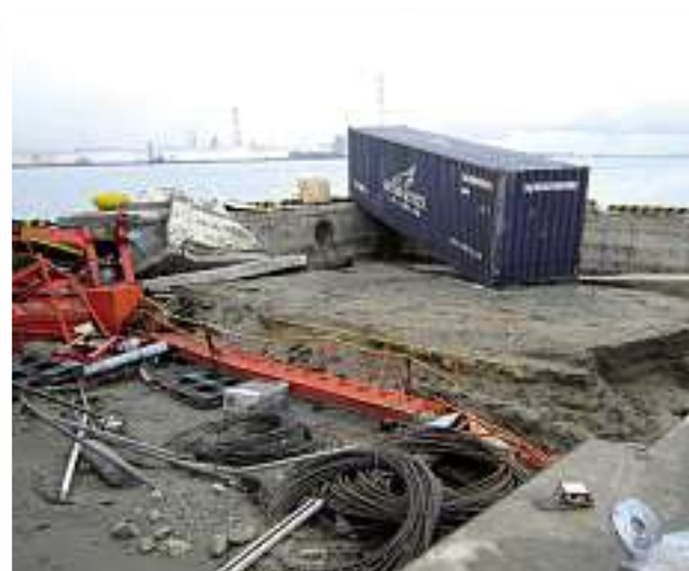
Quay wall at Port of Sendai after the tsunami hit
