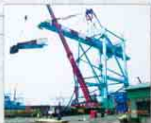
India Crane outreach increased with 3-meter boom extension
