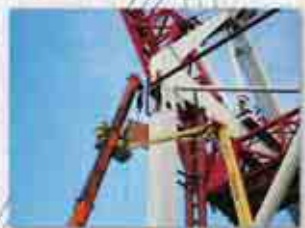
France Repair of crane leg after vessel strike
