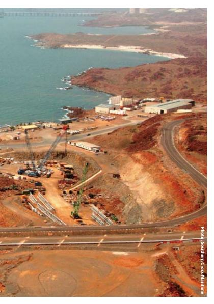
Dampier: one of the Western Australian ports that are receiving billions of dollars to expand Panamax bulk carriers at a proposed new multi-user minerals berth at Utah Point. The project would cut a berth pocket 300m long by 60m wide and 14m deep. The new berth, which would have an initial capacity
