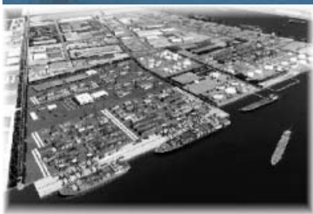
Deep-water container terminal being constructed at Tobishima Pier (to be completed in FY 2005)
