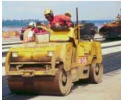
Workers complete upgrades to the Port of Tacoma's North Intermodal Yard
