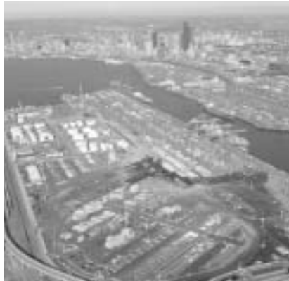
Terminal 18 (Courtesy of Mr. Don Wilson, Port of Seattle)
