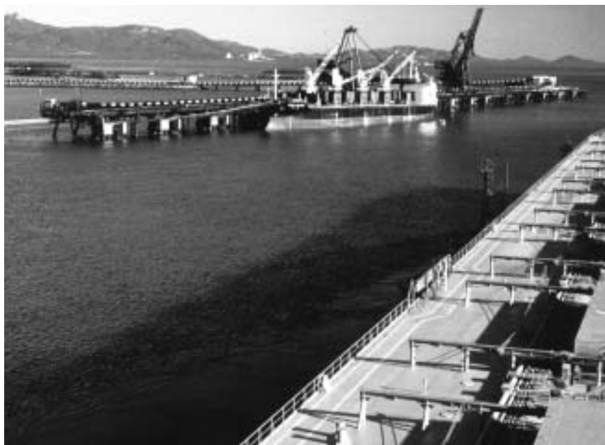
The RGCT Expansion Project will increase the capacity of the terminal from 30 million tonnes per annum (Mtpa) to 40 Mtpa.
