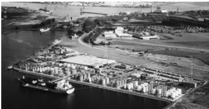
ADPO will invest BFE 1.2 billion (€29.75 million) in a new tank farm and jetty.
