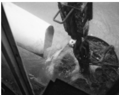
Pennine's Aquacaster system used to combat potential seismic damage in Greece. Picture shows the marine vibropiling hopper being lowered to the sea bed.
