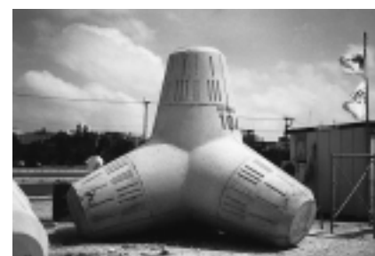
Example of ragged concrete blocks
