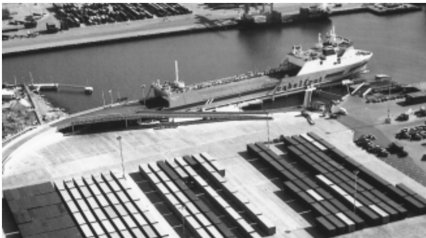
The Paper Terminal at Göteborg's Älvsborg Harbour is designed around the 'secu', the unique cargo unit used for the Sweden-to-Continental Europe paper flow of paper producer Stora Enso. The 80-tonne loads are handled by custom-built straddle carriers and extra strong tractors on a concrete yard and using a triple-ramp system.
