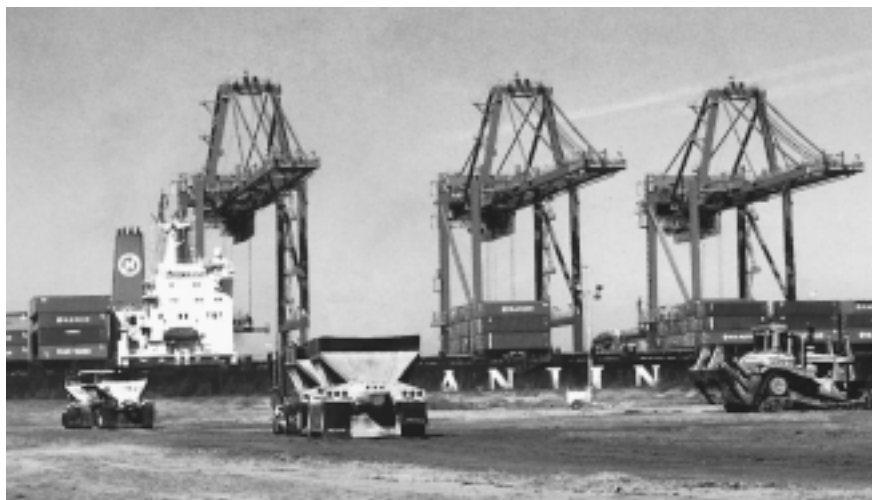
Trucks deliver soil to Pier S for the port's soil remediation project. About 700 trucks deliver an average of 15,000 tons of clean soil to the site each day.
