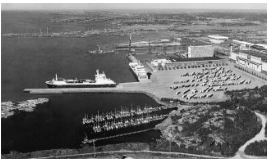
The Arendal project will result in two ro/ro berths to be ready for use by the end of 2000. This phase of the project comprises an 87,000m 2 handling area and the dredging of 80,000m 3 . The Arendal Terminal is being built on former shipyard land.
