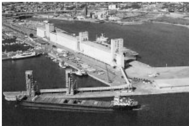
Infrastructure improvements are being undertaken at wharves in the Estuary Sector and the Anse au Foulon Sector
