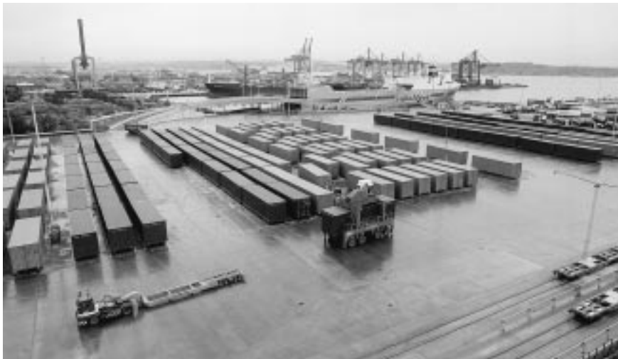
The new Paper Terminal at Göteborg's Älvsborg Harbour is dedicated to the flow of paper from Stora Enso mills in Sweden to Continental Europe markets. Volume not taken up by paper is being used by Cobelfret for Göteborg-Zeebrugge v.v. Shipment. Note the special box and the heavy-duty equipment used to handle the 90-tonne boxes.
