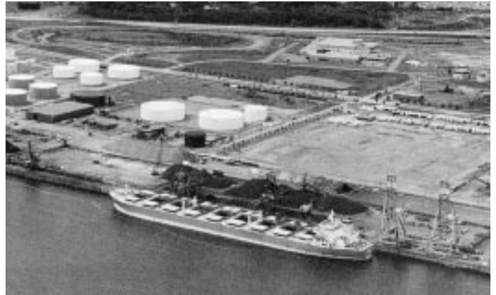
St. Lawrence Stevedoring recently acquired tow gantry cranes
