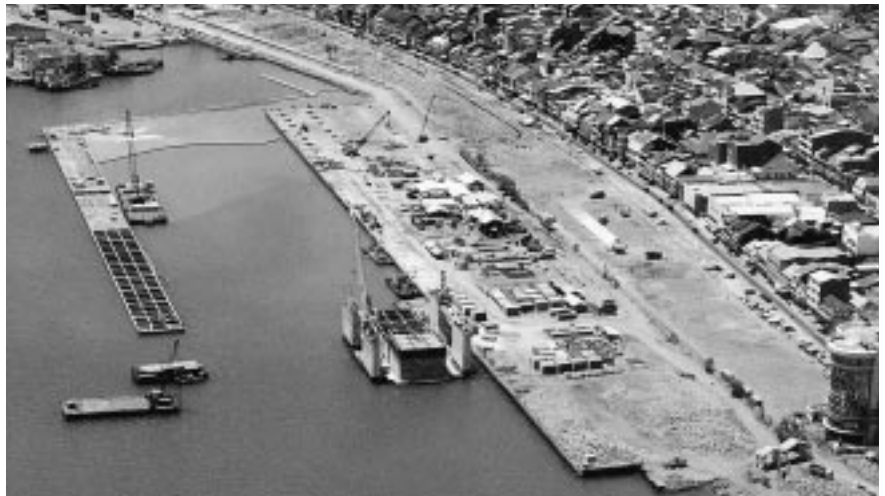
Ujung Pandang Port's urgent rehabilitation project under construction (Indonesia)
