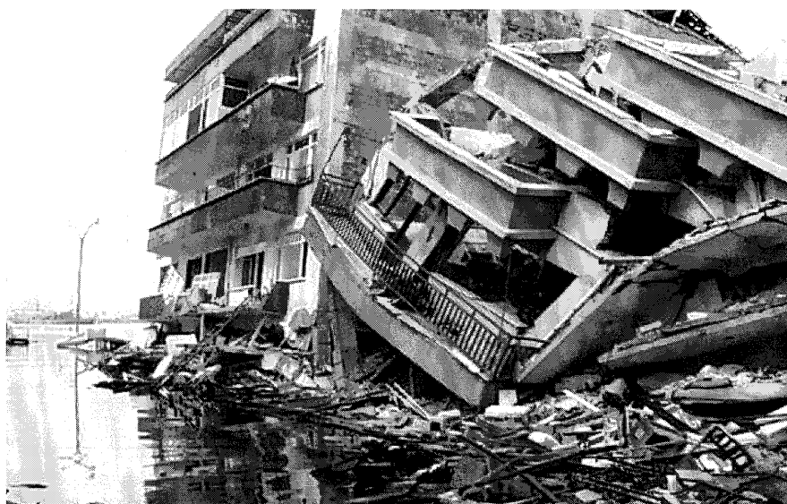
At Golcuk collapsed building and sinking of the road (in front of the building)
