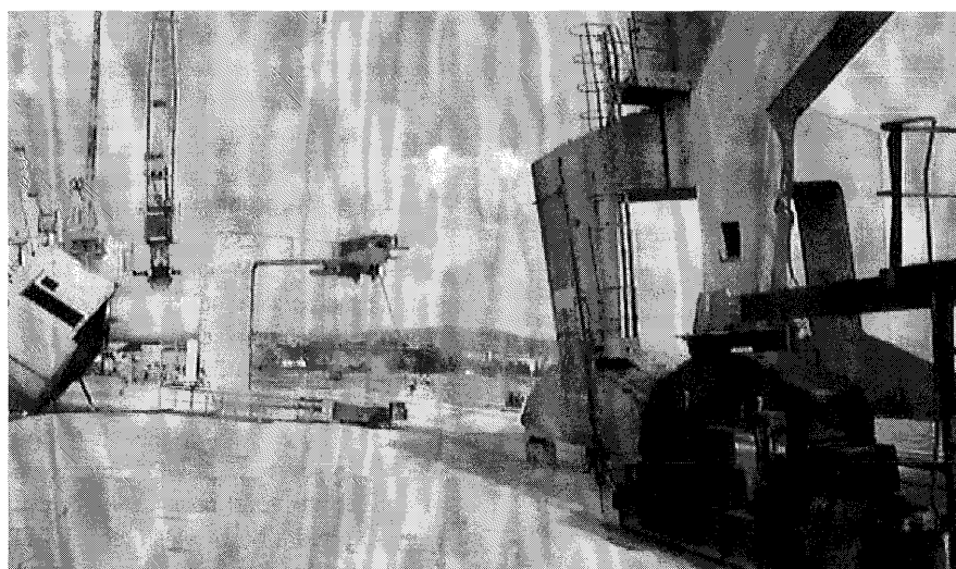
No. 6 Berth at Derince: Collapsed crane, derailed crane, signs of liquefaction, cracks and sinking of concrete slabs
