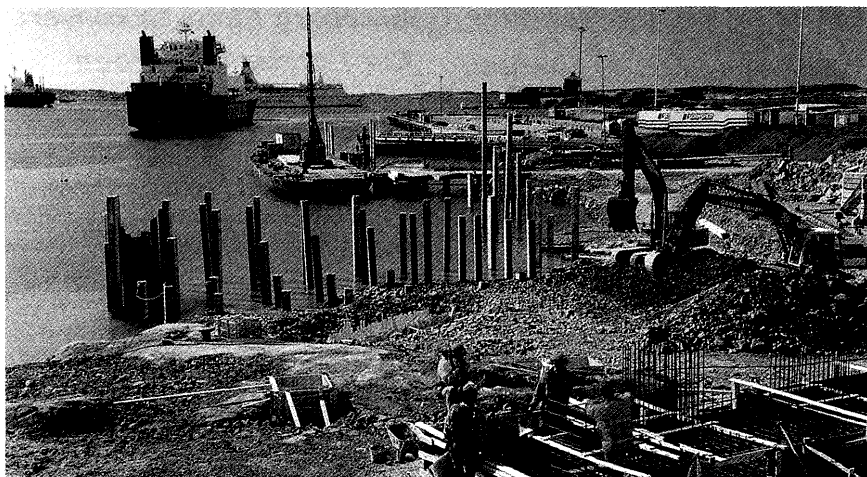
Work is now going ahead on the Port of Göteborg's Berth 700 construction. The berth will handle paper shipments for Stora Enso and also general cargo for Cobelfret. The technique used will have some extraordinary elements. Two-level ro/ro ramps and 90-tonne load weights are two of them, a 53,000-sq-m concrete yard surface is another. (May 1999)
