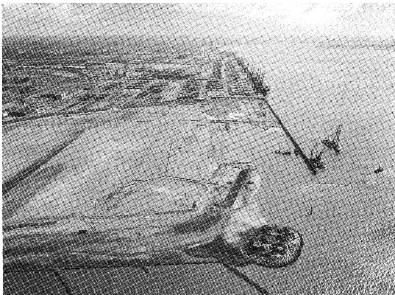
To meet the growing container traffic in Bremerhaven, the River Quay is being further extended to the north. Up to now the total of 700 meters have been completed.
