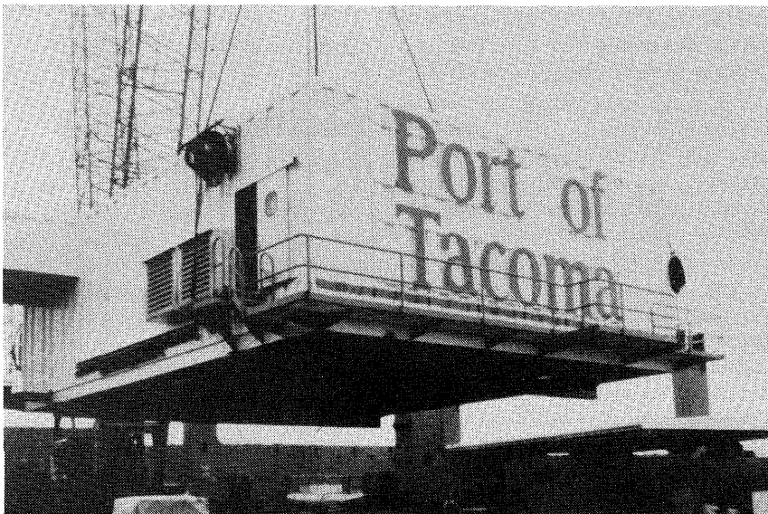
One of the crane housings of the Port of Tacoma's two new container cranes is off-lifted from barges at the newly-constructed Terminal 3.
