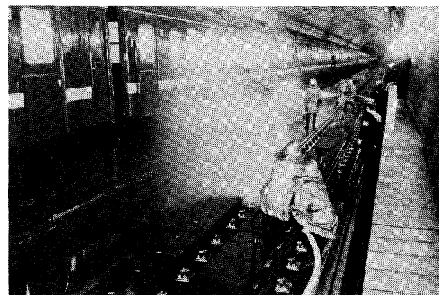
Fire-fighting drill at one of the two stations (emergency stop zones) in the tunnel. A narrow side-walk is situated on both side of the tunnel for letting off passengers. (Picture: Courtesy of Japan Railway Construction Corporation)
