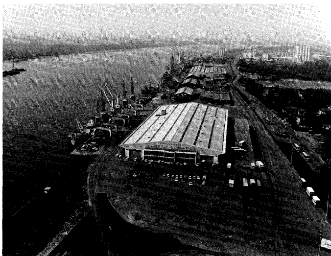
No. 4. This air conditioned shed at BASSENS is served by a double berth for reefer vessels and an axial ramp ro-ro pontoon. On the doorstep of Bordeaux, it serves not only for storage, but as a veritable market for early vegetables and citrus fruits etc. Beyond are the quays catering for containers, oilseed cake and fertilizers and in the distance, the grain terminal with its vast storage silos.
