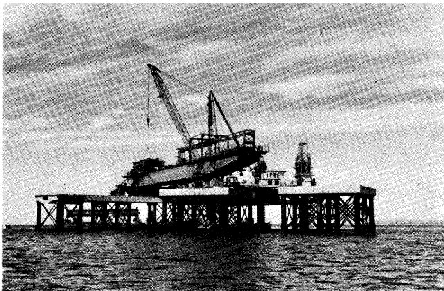
Figure 11—Erection of Slewing Shiploader
