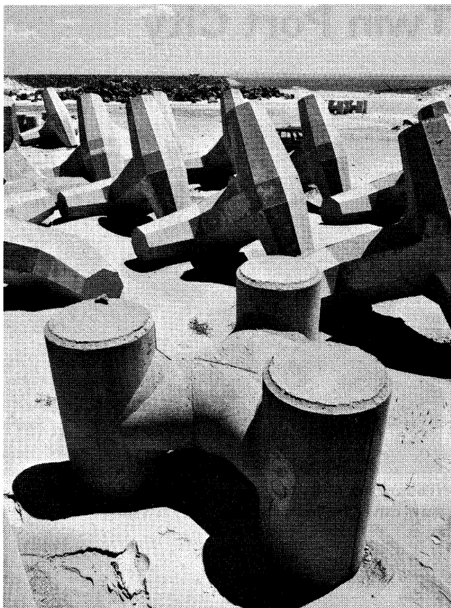
(Photograph C—Tribars and Dolos) The 20 tonne armour unit in the foreground is 2.2M high. The 13 tonne dolos units in the background are 3.3M overall length with 3.3M long flukes.
