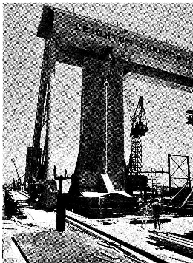
(Photograph F—construction of counterfort units) Construction of 360 tonne, 18.7M (61.4FT) high concrete counterfort wharf units.
