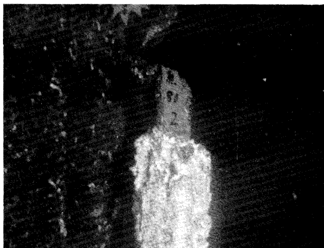
Photo 6. Aluminum Alloy Anode Five Years After Completion of Seabirth
