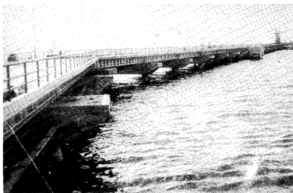
Oil Unloading Pier protected by Cathodic Protection
