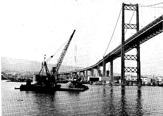
Los Angeles, Calif., 121075 (Port of Los Angeles):—Rock barge unloading continues on Main Channel of Los Angeles Harbor where, seven fathoms down, 100 tons of newly-installed 30-inch sewer main receives an 8-foot protective rock coating to complete Channel-crossing of Board of Public Work's new San Pedro-to-Terminal Island sewer line.
