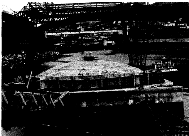
Figure No. 6 The 13.7 m diameter caissons, to be installed at a minimum water depth of 27.5 m, are fabricated with domed bottom.
