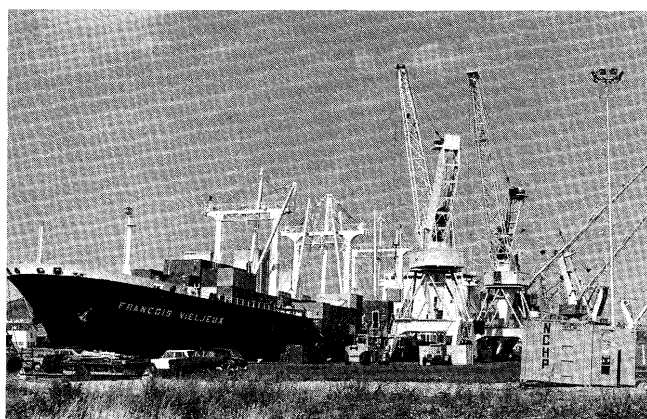
Rouen:—The Rouen Quevilly Quay with containers. At this quay containers are handled with two cranes of 25 tons lifting power each. (Port of Rouen Authority)
