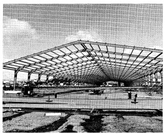
Wellington, New Zealand, 17 June, 1975 (Wellington Harbour Board):--The 2 berth, 12 hectare Thorndon container terminal has fully integrated back-up facilities including sub-surface power points for refrigerated containers; container washing, dangerous goods and break bulk depots. Picture shows new break bulk depot under construction with gross floor area 9,451.32 m<sup>2</sup> or 231.65  $\times$  40.80 m.
