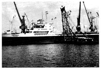
**PORT OF HELSINGBORG** Heavy lifts at Helsingborg are now performed by a floating crane with a lifting capacity of 200 tons—here doing service at the Ocean Terminal.
