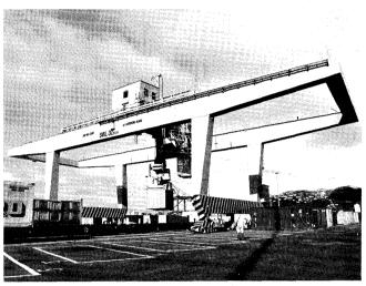
PORT OF WELLINGTON-RAIL TRANSFER CON-TAINER CRANE: The Rail Transfer Terminal Crane is used for lifting containers on to or off rail wagons
