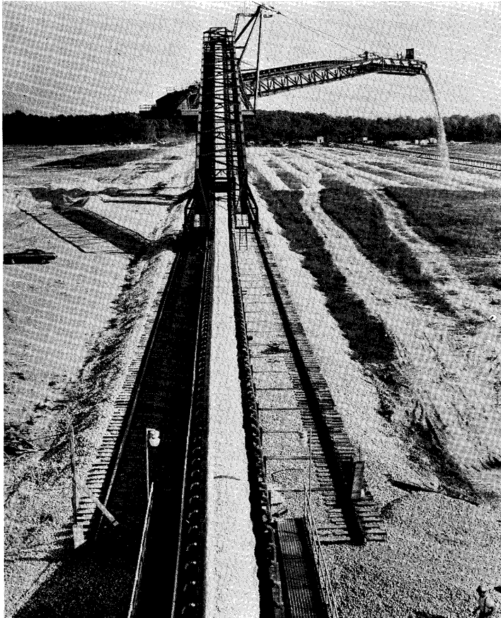
Figure 5:—Crushed stone for storage yard base was received in ship-loads and spread by the stacking system.
