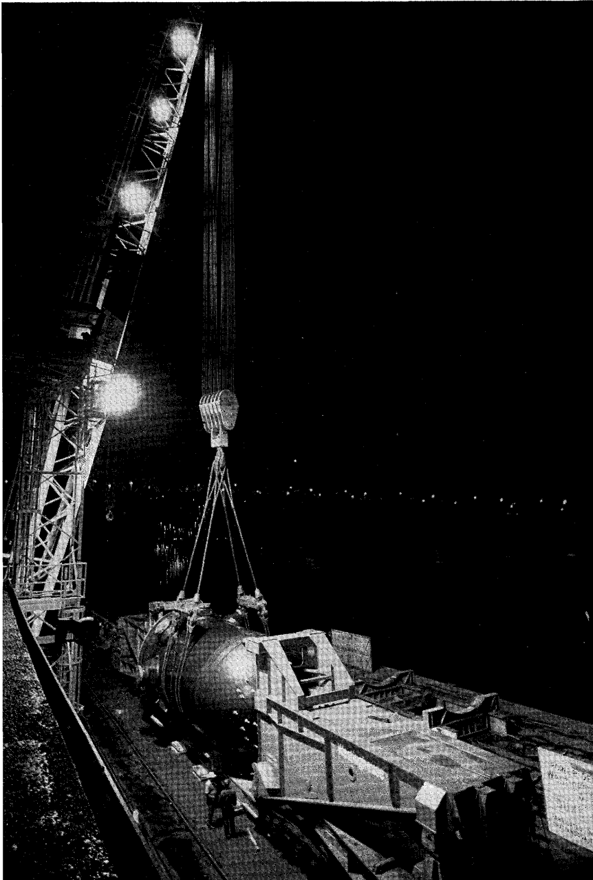
RECORD LIFT —The South Carolina State Ports Authority's 400-ton crane, known affectionately around the Charleston area as "The Monster," made an SPA record lift recently when it hoisted this 370-ton nuclear reactor vessel from a barge to a waiting custom-built flatcar. Believed to be the heaviest piece of equipment ever lifted by a fixed dockside seaport crane in the Western Hemisphere, the reactor vessel was built by Combustion Engineering, Inc., of Chattanooga, Tenn. The giant component, headed for its installation site at a Duke Power Co. plant near Charlotte, N.C., was brought by barge to Charleston because the port has the only crane on the U.S. Atlantic Coast that could handle the load. (December 12)
