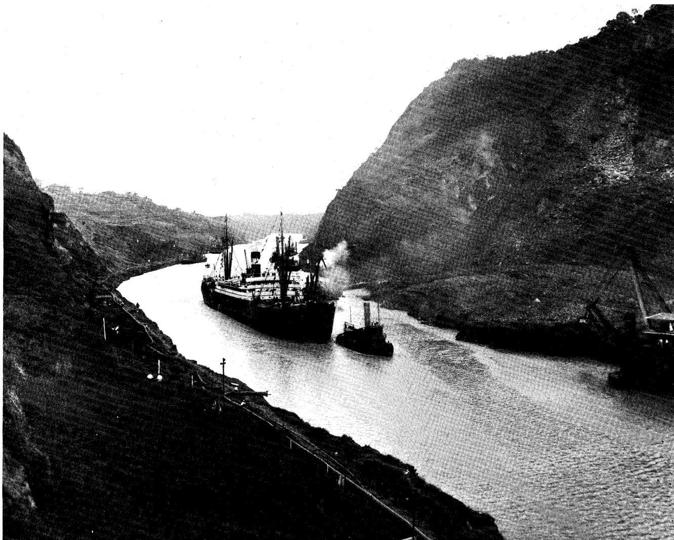
Officially opening the Panama Canal, August 15, 1914, the old SS "Ancon" passes a slide in the area now known as Gaillard Cut. Since mud and rocks were still sliding into the Canal, the "Ancon" was a rather snug fit in the channel. It was here that the devastating slides occurred during construction days.
