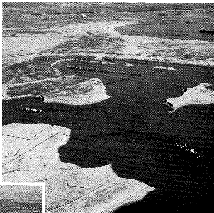
11 Adriaan Volker dredgers making new harbour basins for Rotterdam
