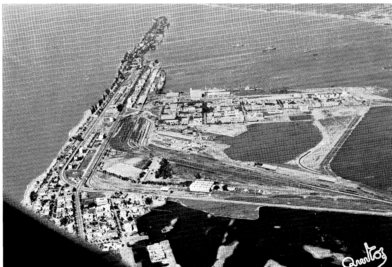
Aerial view of Lobito Port
