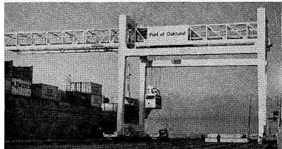
LOW PROFILE PORTAINERS meet height restrictions and cover more yard area
