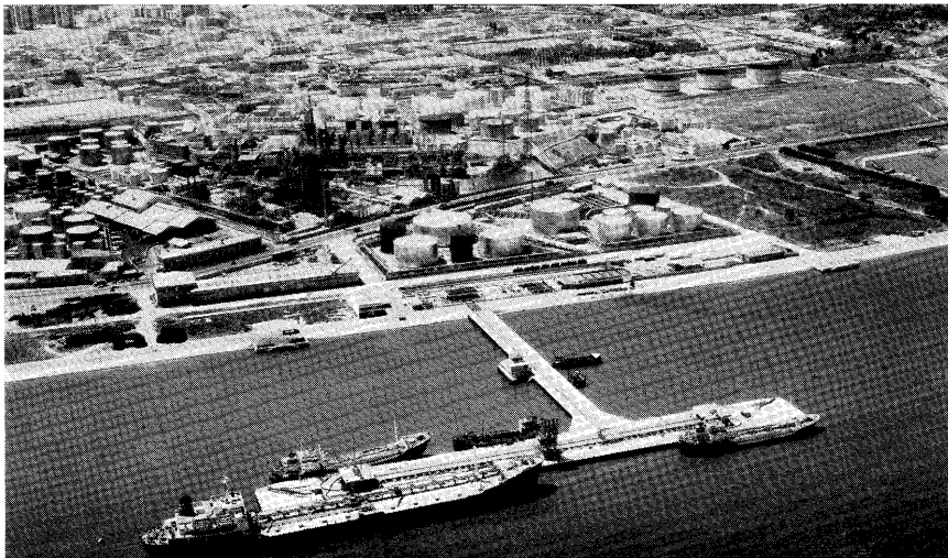
Cabo Ruivo pier-bridge, serving the terminal for oil tankers, up to 65,000 tons.
