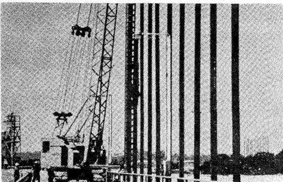
Reconstruction work in progress using BHP steel H piles at No. 1 Kwinana jetty.
