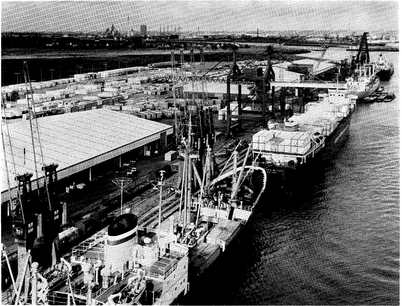
The Container Terminal Bremen has possibilities both for full-container ships and for semi-container vessels. 800 m quay length, two container bridges and more than 100,000 sqm of marshalling yard. On a 22,000 sqm shed without ramps, port-to-port containers can be emptied or filled. Handling equipment of 6 van-carriers, 7 trucks with a hydraulic fifth wheel, 2 Diesel-fork-lifts with a 5-t-capacity and 9 with 3.5 tons is available.
