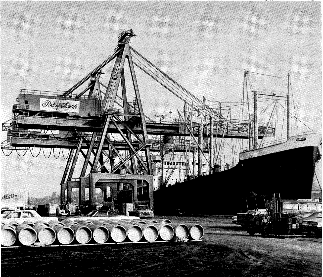
Two Hitachi 30 long-ton container cranes installed at the Port of Seattle, Washington
