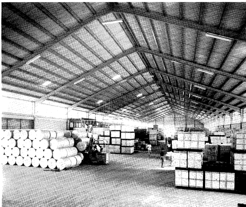
The interior of one of the Port Authority's modern portal-frame structures for covered storage purposes. The Authority has over 1.3 million sq ft of transit sheds, 295,000 sq ft storage warehouses, 218,000 sq ft leased warehouses, and open storage space (concrete surface) totalling 855,000 sq ft. In addition, there are car parks with a total of 66,000 sq ft.—The Port of Singapore Authority
