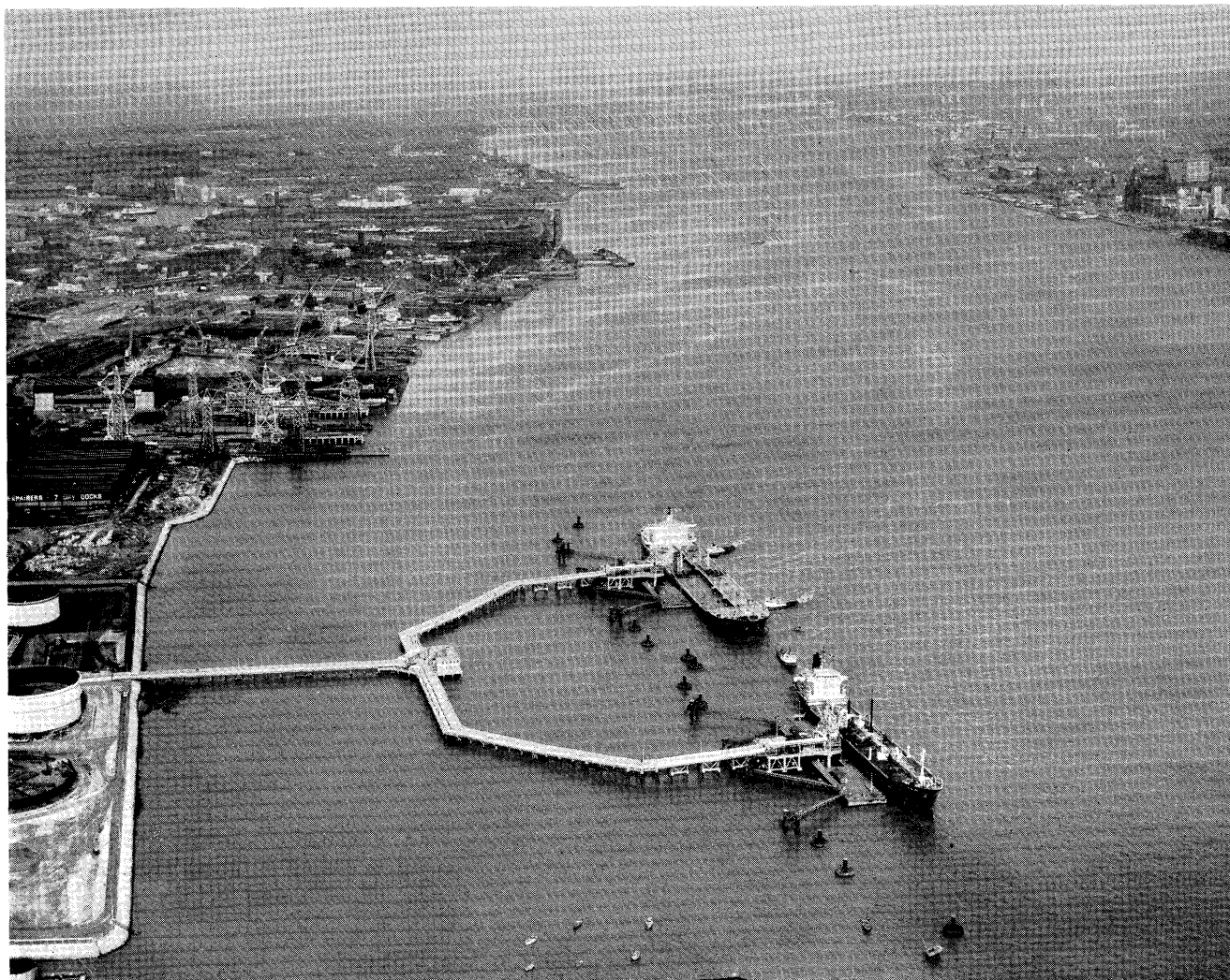
Port of Liverpool—The River Mersey at Tranmere Oil Terminal capable of dealing with 200,000 ton oil tankers.
