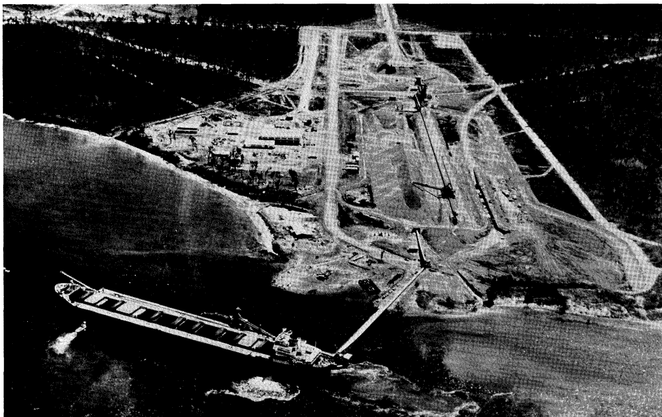
1. The M. V. Siglim of 65,000 dead-weight tons, berthing at the new Lorim Point Wharf at Weipa to load bauxite from stockpile. The bauxite is mined in the area in the background.
