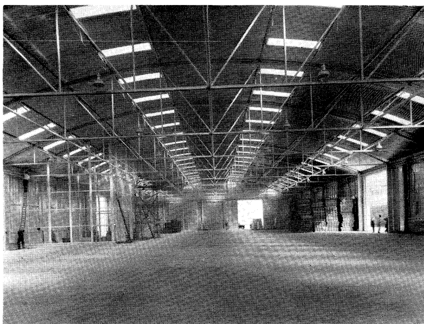
Interior View of "G" Shed, Millwall Dock, one of the most modern erections in the Port of London, and part of a major development on the west side of Millwall Dock. Constructed in tubular steelwork the shed is 350 ft. long and its roof is supported by bowstring girders of 150 ft. span, 21 ft. 6 ins. clear above the floor, thus affording ample space for the use of modern mechanical equipment.
