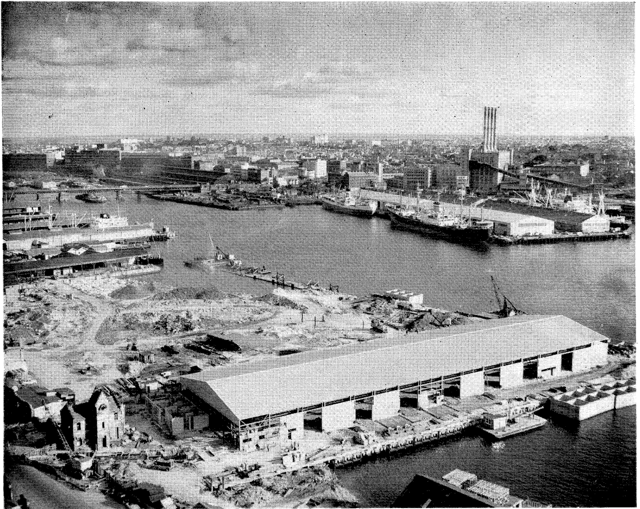
Work is well in hand on the remodelling of wharfage in the Darling Harbour area of the Port of Sydney. One of the new structures will provide accommodation for up to five overseas vessels with wide cargo sheds and ample areas of open space for the storage of cargo not requiring coverage.
