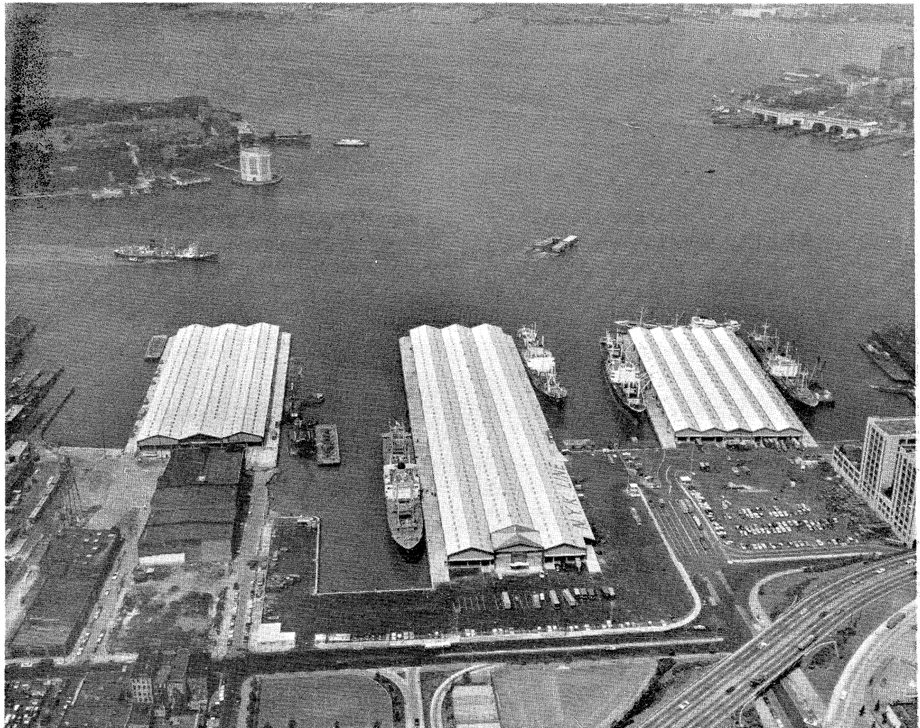
Three Piers recently completed by the Port of New York Authority along the Brooklyn Waterfront have extensive upland areas and wide aprons.
