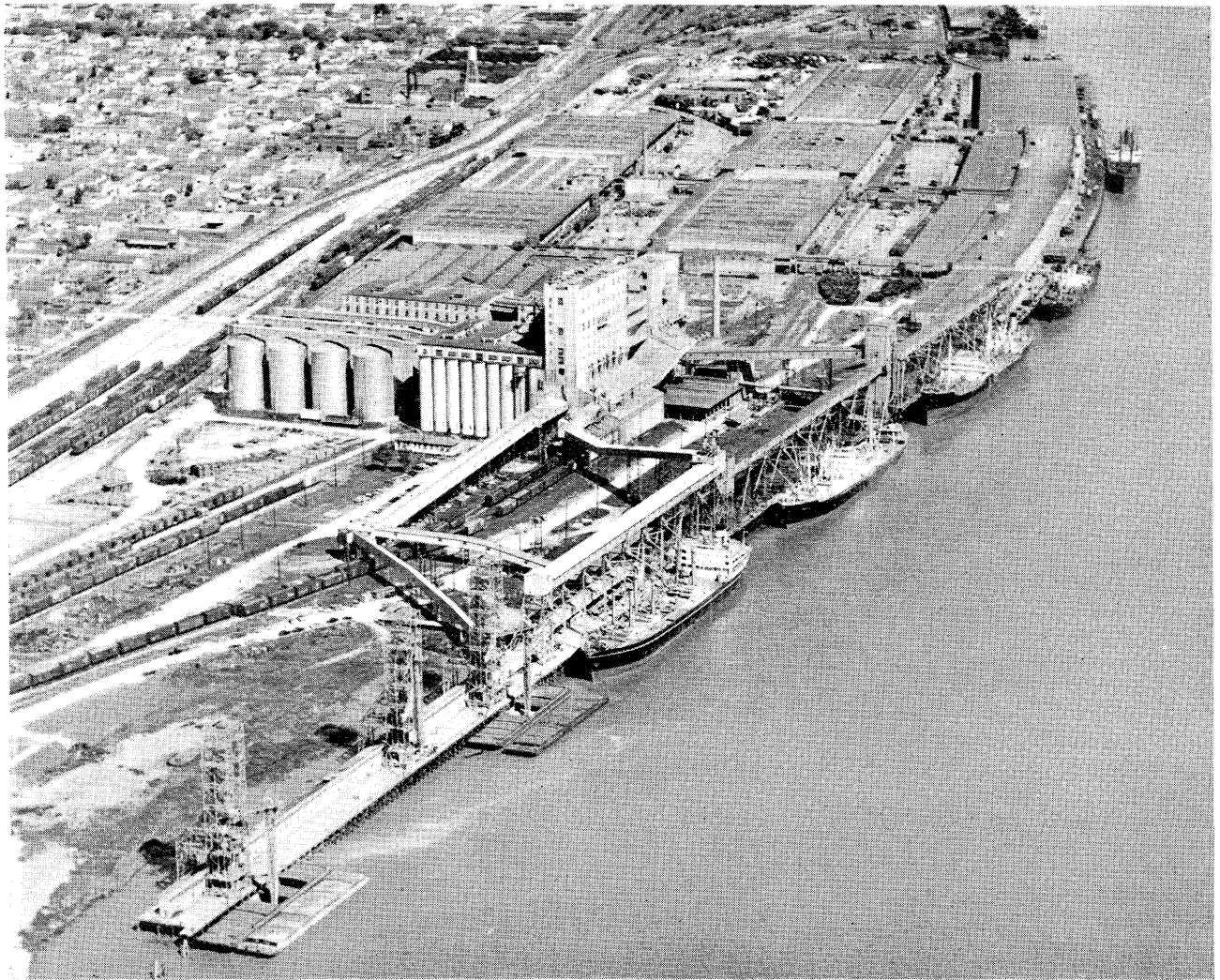
The Public Grain Elevator at New Orleans is now capable of turning over a million bushels of grain every work day. Three ships can outload bulk grain and one sacked grain simultaneously; barges can be unloaded at three mobile marine legs, at the rate of up to 12 per day. Rail cars unload at the rate of one almost every five minutes.
