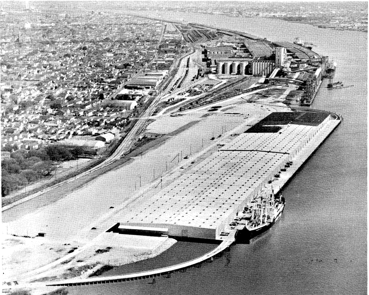
The new Nashville Avenue Wharf at the Port of New Orleans is shown as it was first placed in use recently. Its 2400 feet of water frontage accommodates four ships, which can load and unload simultaneously, as well as exchange cargo with over 100 rail cars, 64 giant trucks and barges. In the background is the giant Public Grain Elevator.
