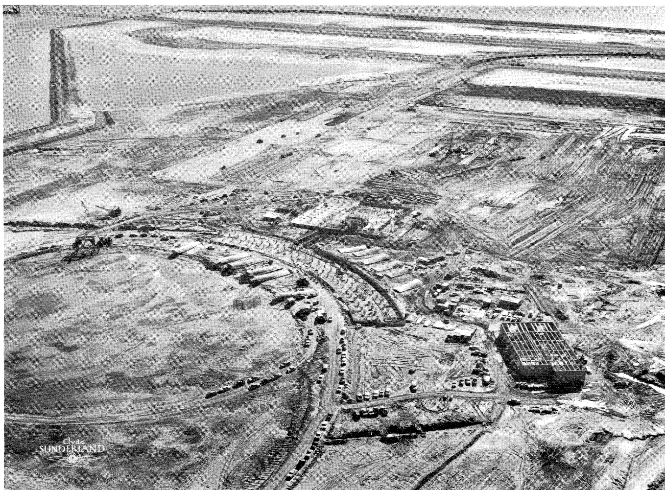
Construction of the passenger terminal and other improvements from approximately the same angle as the artist's drawing, shows the parking lot, ticketing building, lobby and finger, with part of 10,000-foot runway at top. The expansion will be completed in 1962.
