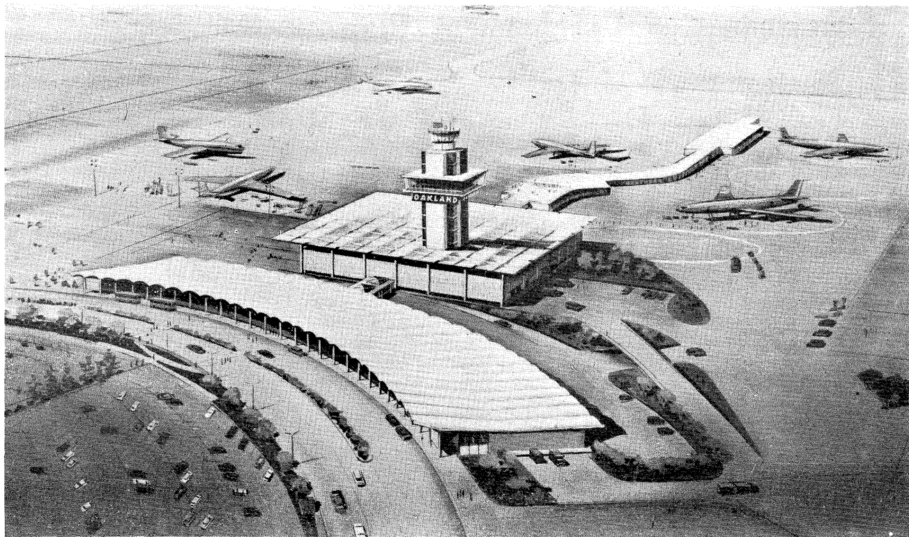
This is an artist's drawing of the new $5,200,000 passenger terminal under construction at Metropolitan Oakland International Airport. Shown are a portion of the parking lot, the curved, canopied ticketing building, the lobby and eleven story control tower, and finger.
