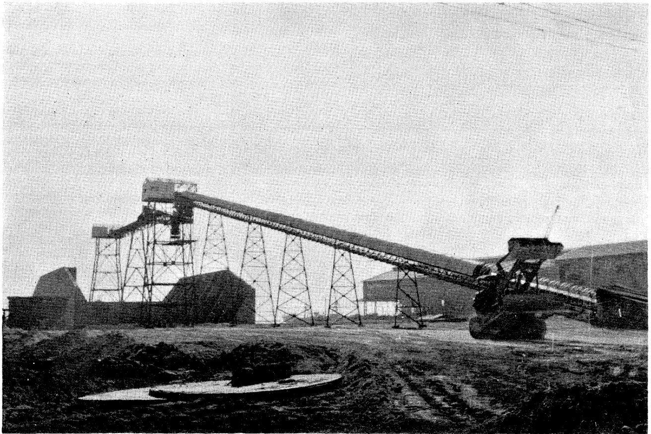
Terminus of belt-conveyor, with the stockpile underneath.
