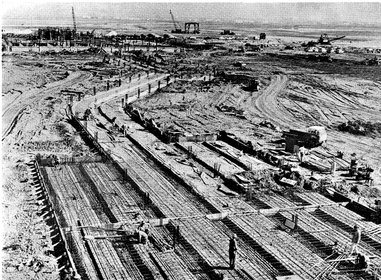
This is part of the passenger loading finger, a dog-leg structure, looking toward the main terminal lobby. Widened portion at bottom is for holding rooms, where passengers will wait to board their planes. The finger will have gate loading positions for 10 aircraft simultaneously.
