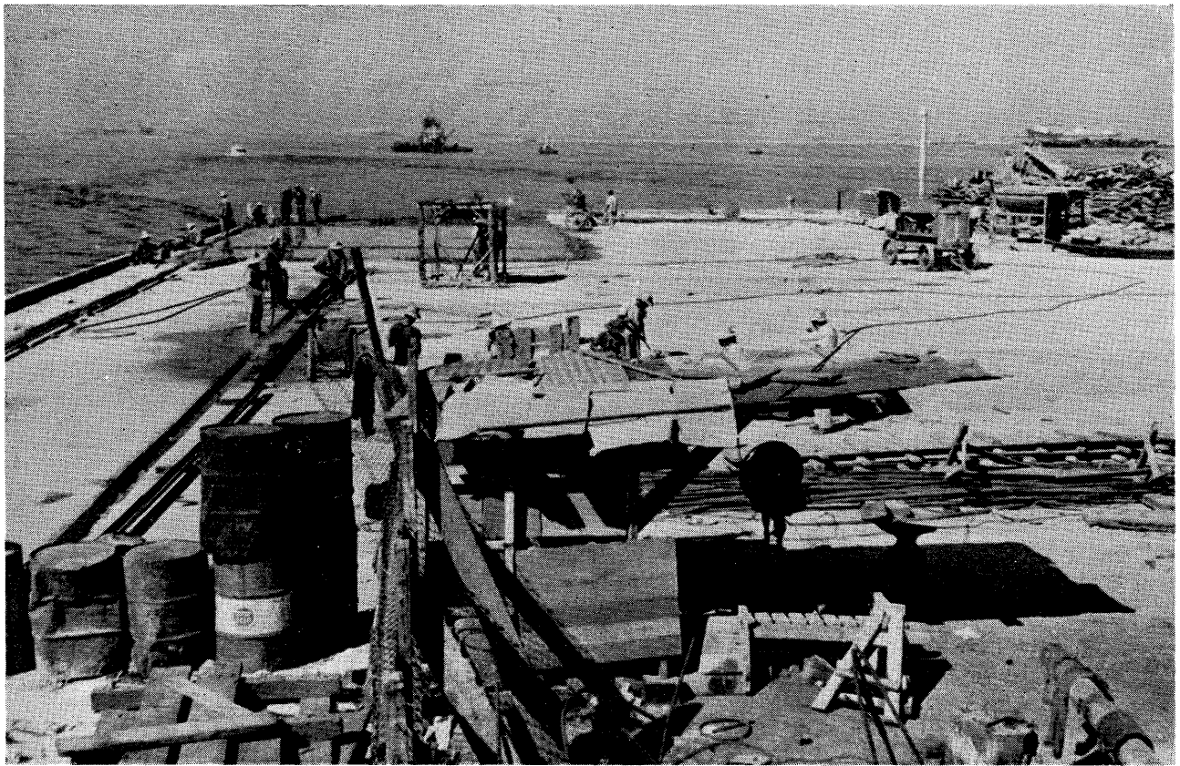
Photo above shows lengthening of Pier 9 in the Port of Manila. The project financed jointly by the ICA and the Philippine Government is expected to be completed soon. When completed Pier 9 can accommodate six large ocean-going vessels at one time.
